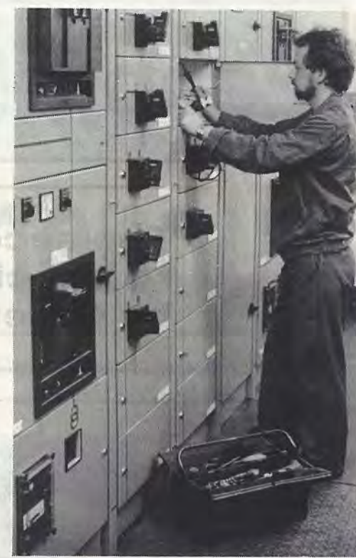
Above: North Wirral based Contracting Electrician Derek Povall tests the supply on the out-going breaker at British Leather.
